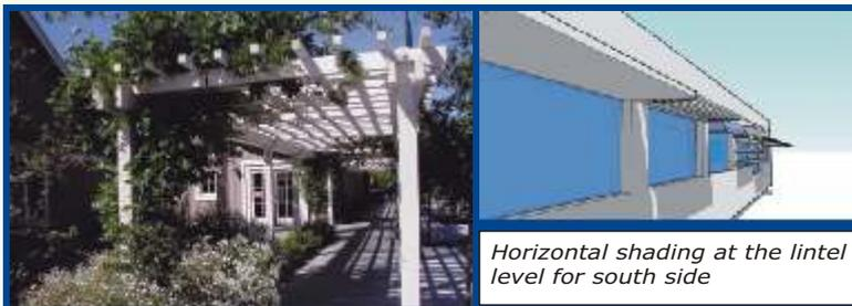
allowing them in during winters. This helps protect the building from over heating during summers, and keeps it warm during winters, thereby reducing the electricity consumed by room coolers/heaters. Windows on the east, west, and south of the house should be adequately protected by *chajjas* and sunshades. In case such features are absent, provide awnings or other shading devices to protect windows from direct sunlight.
