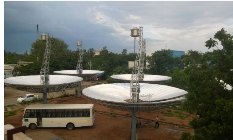
Paraboloid Dishes at Synthokem Pharmaceutical, Hyderabad (540 m 2 ; Process Heating)
