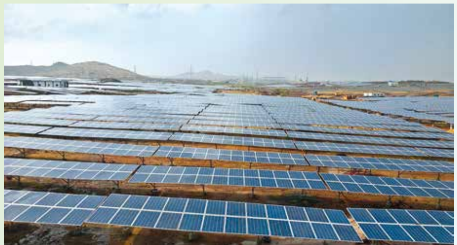
➤ Picture 1: 1,500 MW in Ananthapuramu Solar Park, Andhra Pradesh
