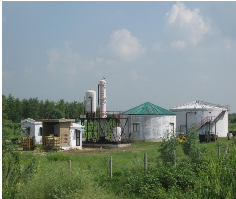
Biogas bottling project of 600 m 3 /day capacity at Anand Energy, Vill. - Kallatiba, Dist.- Ferozepur (Punjab)
