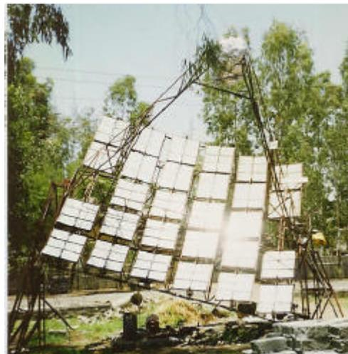
Figure 3 : The Dynamic Fresnel Paraboloid Concentrator with Point Focus installed and tested at Kolhapur– May 1998
