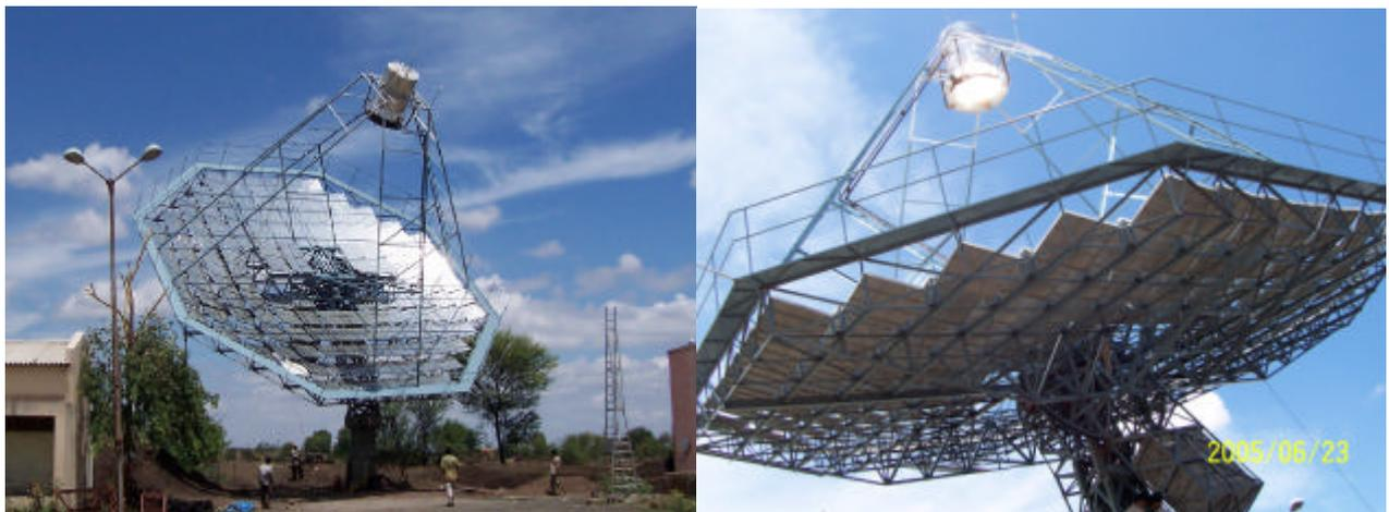
Figure 2 : ARUN160, installed at Latur for milk pasteurisation and its focus on focus plate– June 2005
